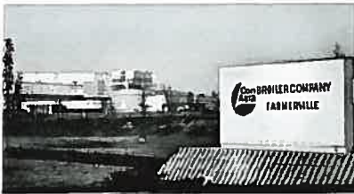
Photo courtesy of Lincoln Builders, Inc.
